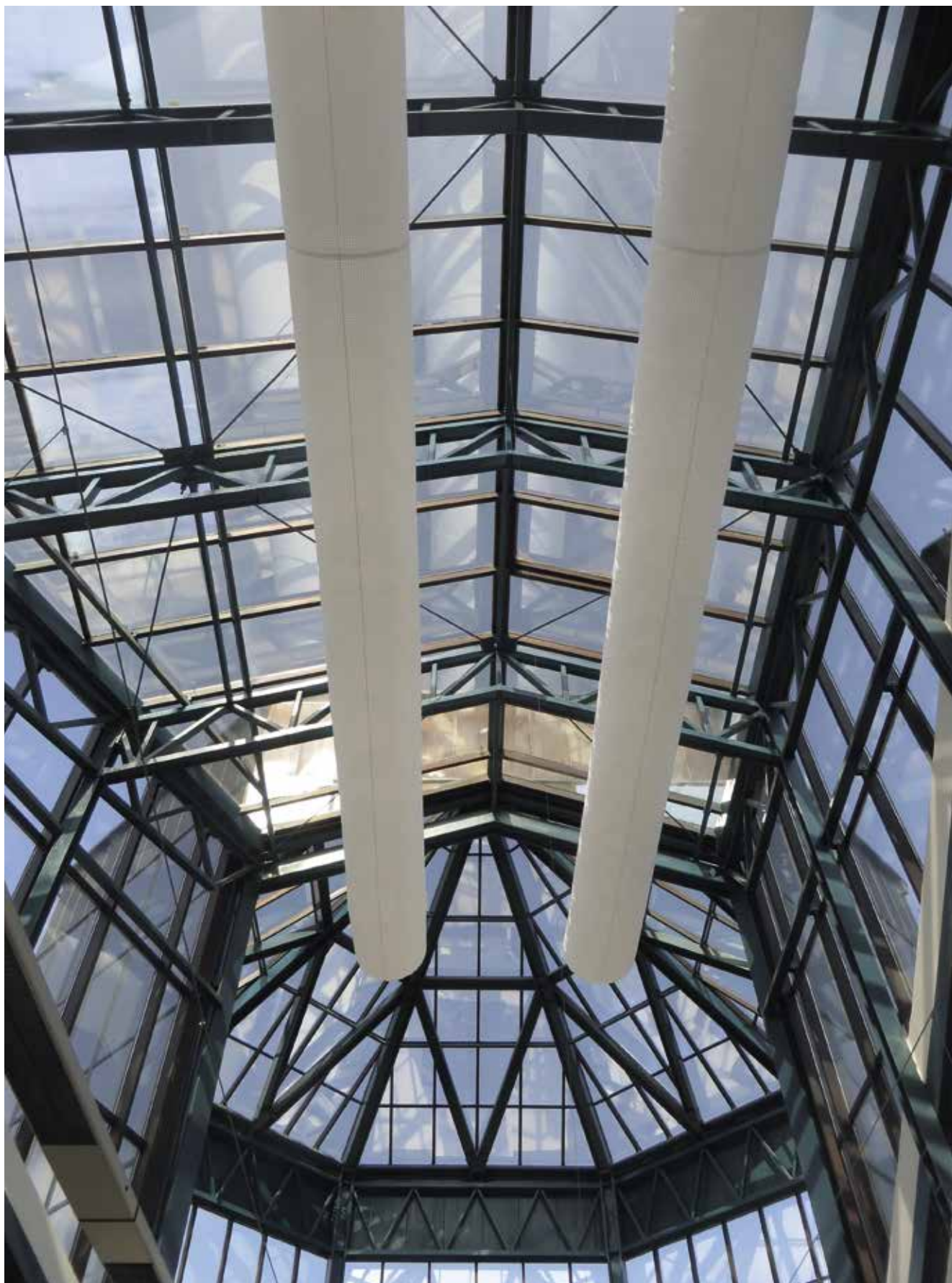
Gaine DHI TEXTILE DHI TEXTILE diffuser
