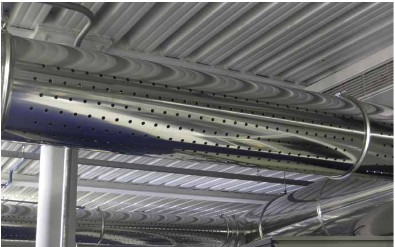
Gaine DHI METAL DHI METAL diffuser
