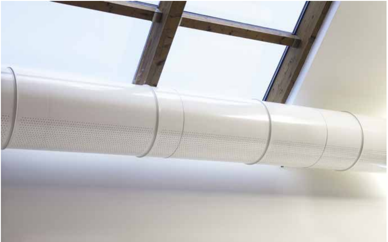
Gaine DHI METAL DHI METAL diffuser
