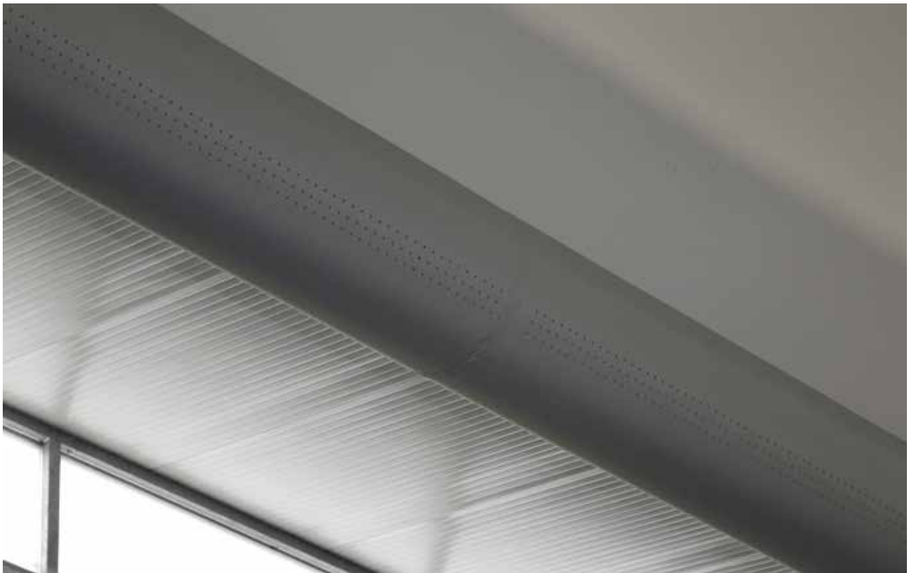
Gaine DHI TEXTILE DHI TEXTILE diffuser
