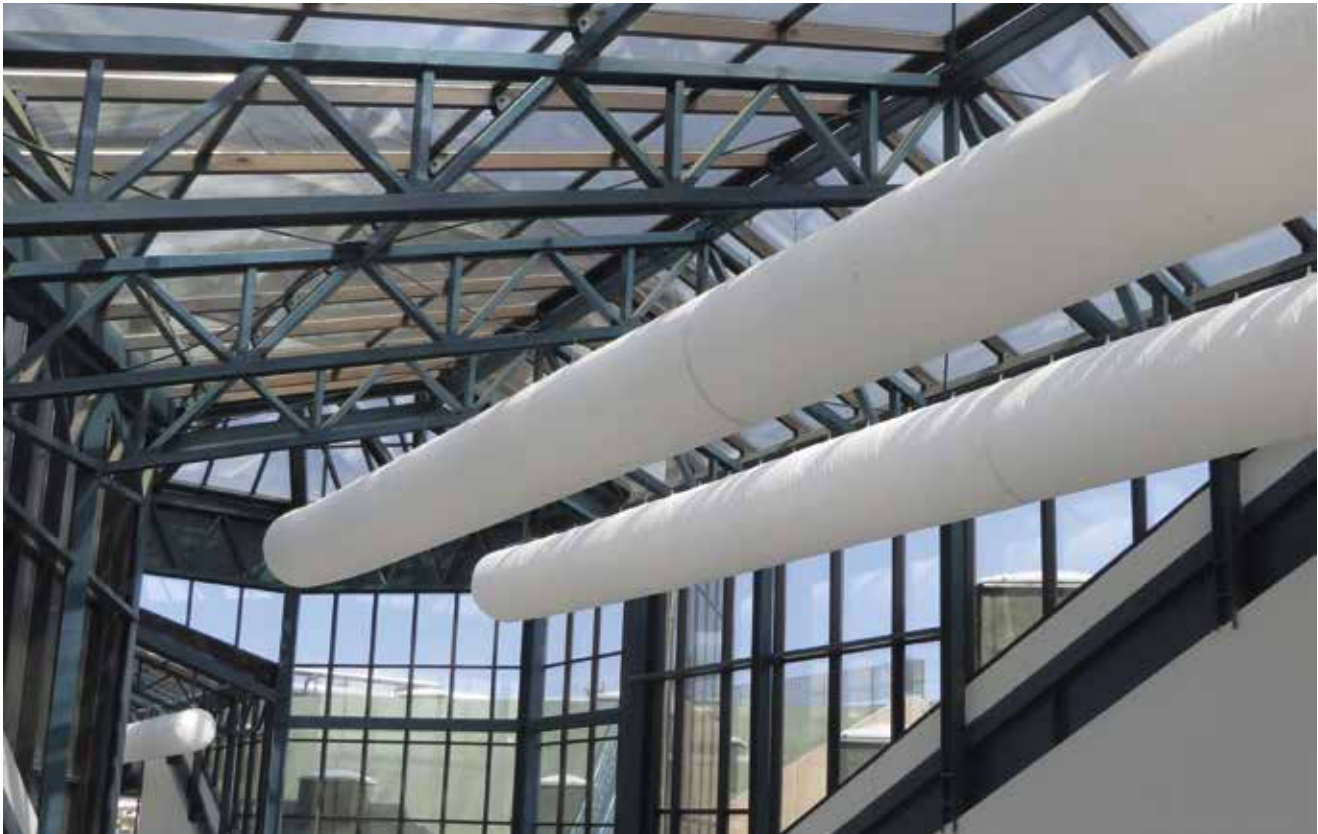
Gaine DHI TEXTILE DHI TEXTILE diffuser
