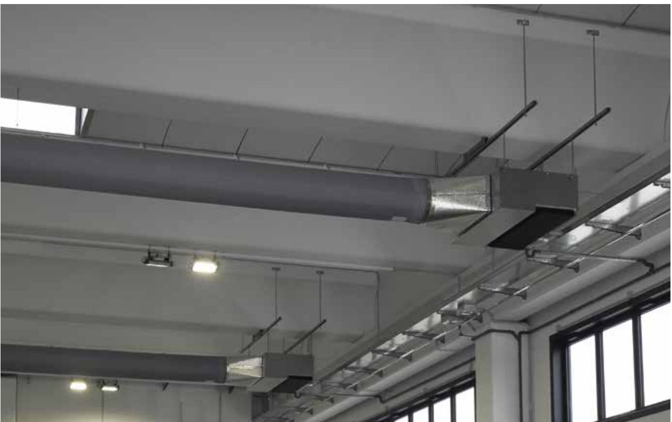
Gaine DHI TEXTILE DHI TEXTILE diffuser
