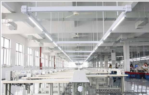
塑管照明配电母线 Plastic-tube Lighting Power Busbar
