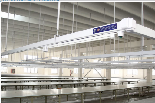
塑管照明配电母线+塑管配电母线 Plastic-tube Lighting Power Busbar & Plastic-tube Power Busbar
