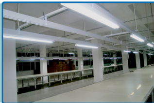
塑管裁剪母线 Plastic-tube Trolley Busbar
