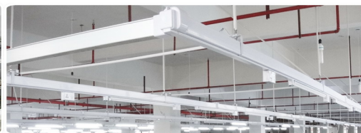
铝合金照明配电母线 Plastic-tube Lighting Power Busbar
