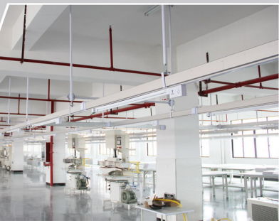
铝合金照明配电母线 Al-Alloy Housing Lighting power Busbar
